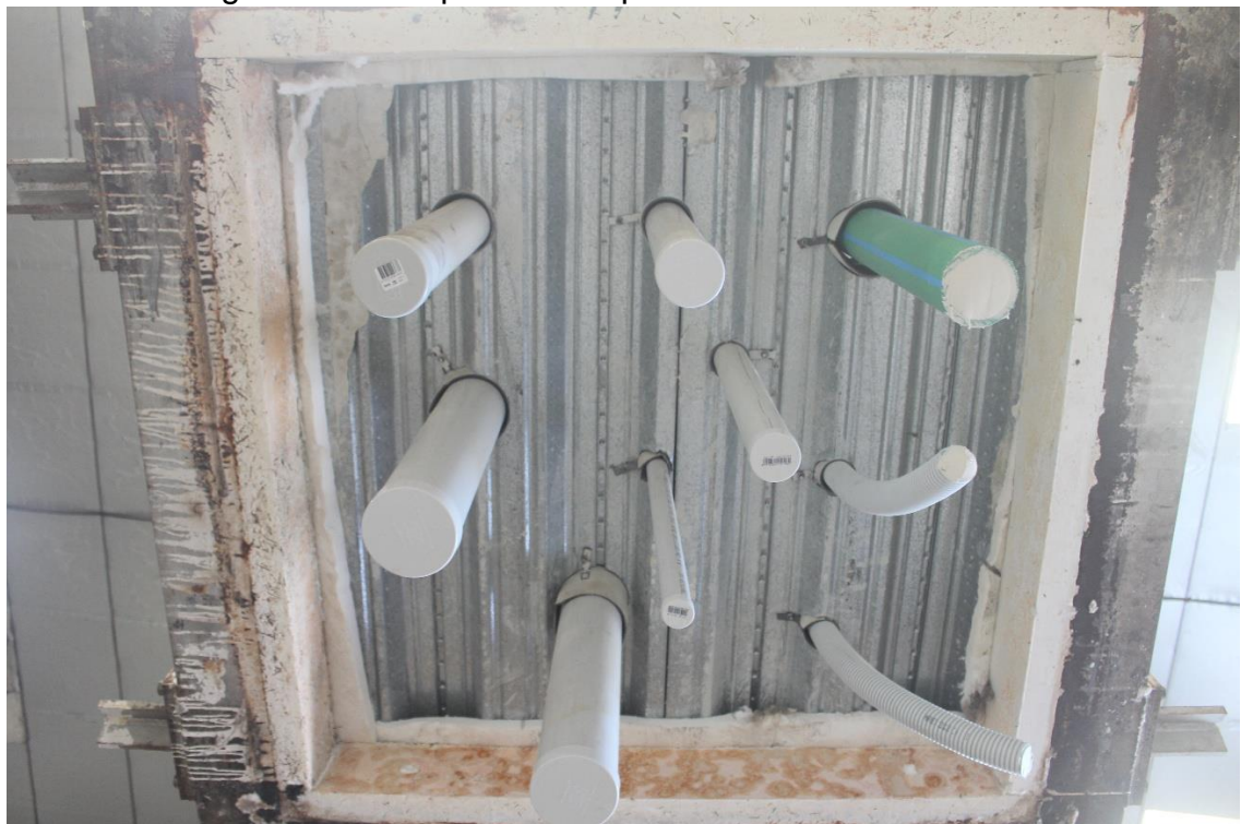
Figure 2 – Exposed face prior to test commencement
